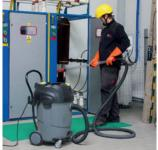
The first of the technologies performed is dry cleaning – by vacuuming and then, as needed, we clean it with the wet method. After cleaning, inspection is carried out with a camera.
